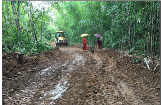
Inspecting the new road leading to Mahabodhi Nobinchera center
