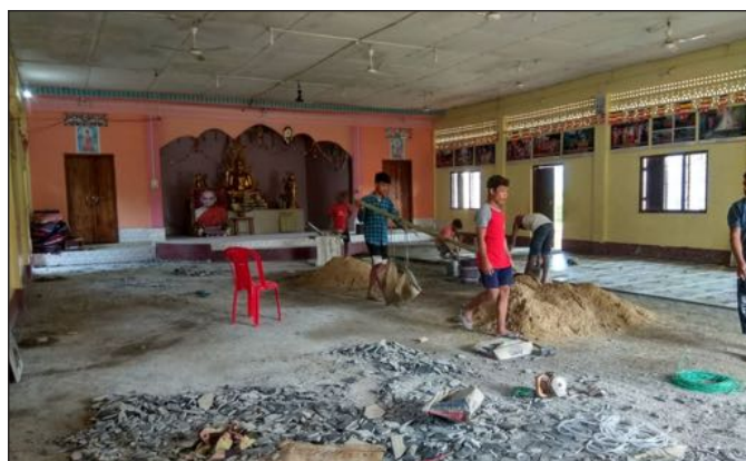
Renovation or the Main temple in progress at Mahabodhi
