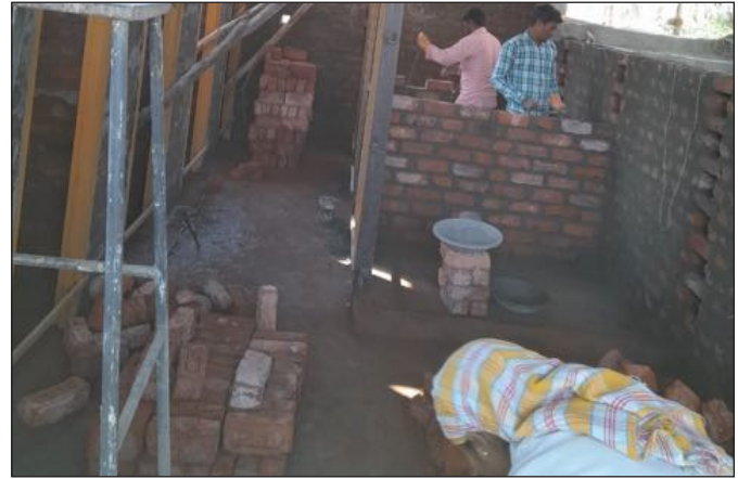
Sangharama monks residence under construction at Mahabodhi center
