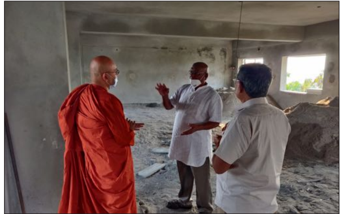
Ven Sugatananda and Mr Anjaneya Reddy inspecting the construction work.
