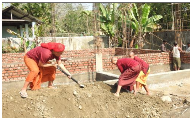
Construction is progress of the dining hall.
