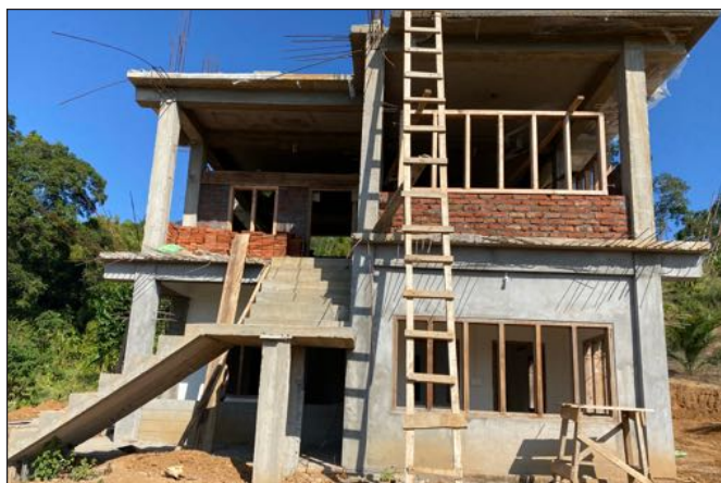
Under construction of Monastic building at Mahabodhi Nongtaw
