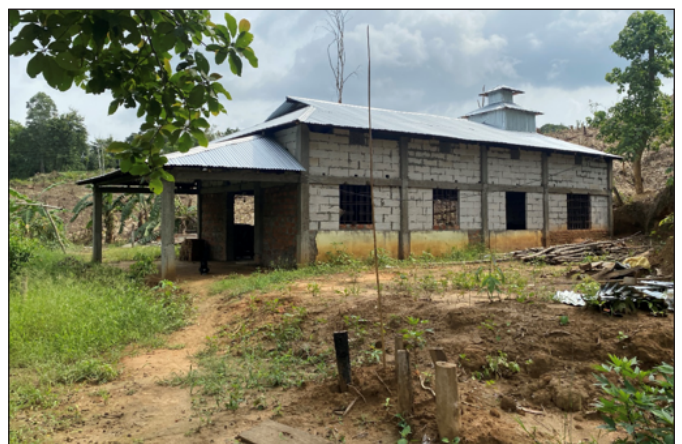
The new under construction at Nobinchera, Tripura
