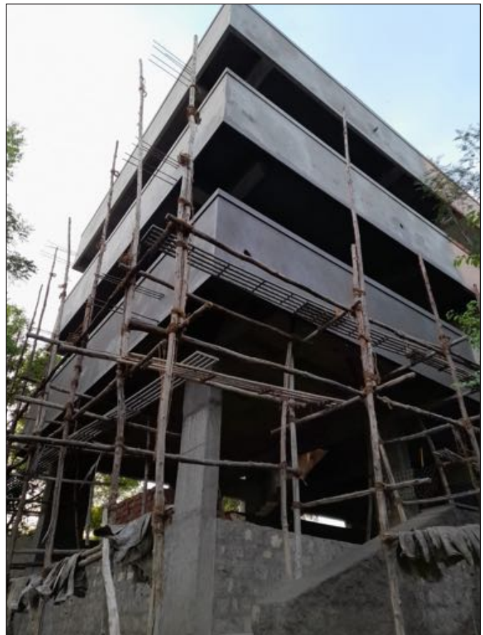
Plastering of the Sangharama building in progress at Hyderabad
