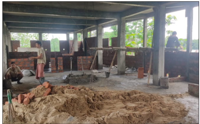
The construction of new hostel building in progress at Mahabodhi
