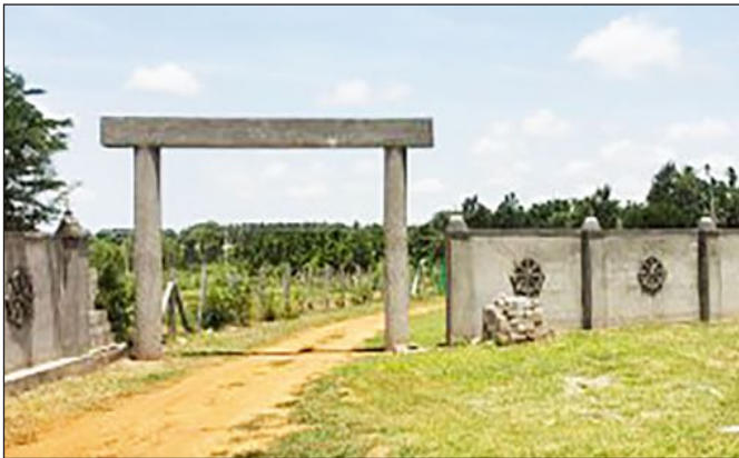
The new gate and extended compound at Mahabodhi Meditation center, Bengaluru.
