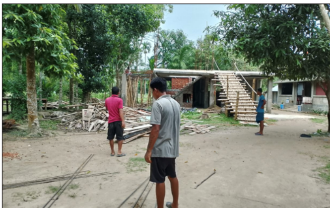
Under construction of dormitory at Harina Mahabodhi.
