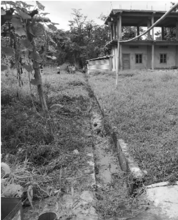
Construction of Drain
