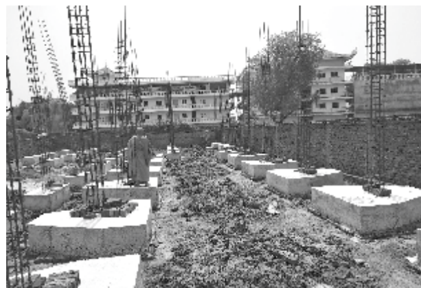
Ven Kassapa Maha Thera inspecting the Construction work of Mahabodhi Bodhgaya
