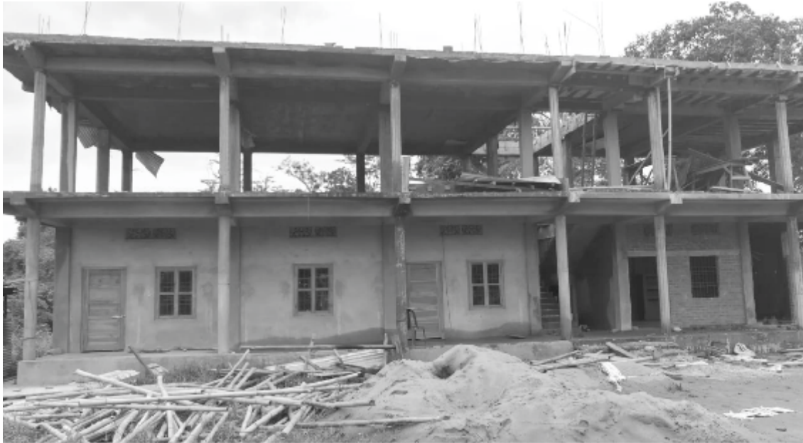
Construction of new Hostel Building
