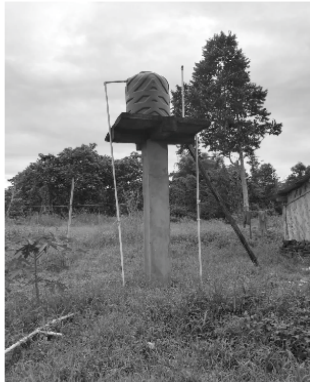
Construction of water tank stand.
